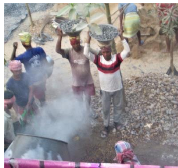
An astonishing precision work from down to above, to fill the mixer, send the elevator, fill up the two wheelbarrows, bring them to the last stretch of armed concrete and come back just at the time to pick the last flow. Not one minute wasted the whole day, except two times for myself. I was very grateful for their satisfied smiles and energy!
