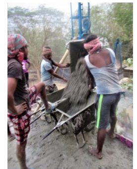
An astonishing precision work from down to above, to fill the mixer, send the elevator, fill up the two wheelbarrows, bring them to the last stretch of armed concrete and come back just at the time to pick the last flow. Not one minute wasted the whole day, except two times for myself. I was very grateful for their satisfied smiles and energy!
