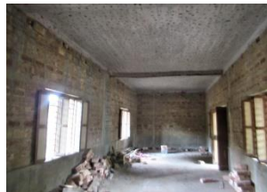
One of the 6 rooms
